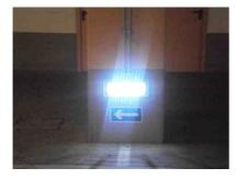
At LoureShopping, emergency lights in the car park area (floors 1 and 2) were scheduled to be replaced in 2011 and the team took this opportunity to retrofit the existing lights with an energy efficient solution. A total of 600 lights were taken out and LED lighting installed, at a cost of  $\in 2,600$ . Each new light, provided by the company Alternative4U, has an autonomous power supply and consumes no more than 3W. The lights can
