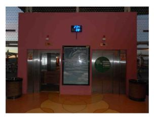
The team identified that lighting was not needed in the shopping centre's lifts when they were not in use, and therefore decided to install presence sensors that would automatically switch the lights on and off. Fluorescent light bulbs were also substituted by more efficient LED bulbs by the maintenance contractor, Schindler.
