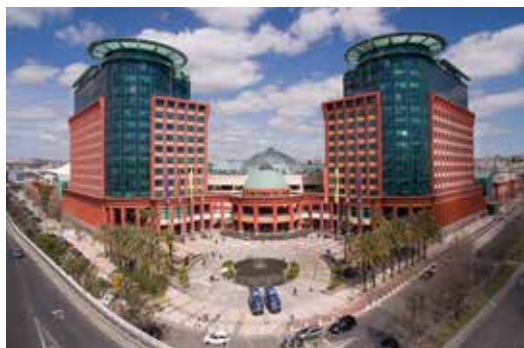
CENTRO COLOMBO TORRE OCIDENTAL AND TORRE ORIENTE · PORTUGAL
